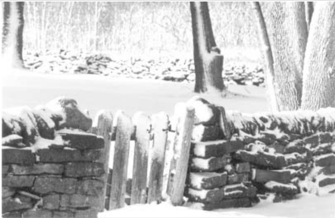
The old gate and fence (at 15095 Front Road)
