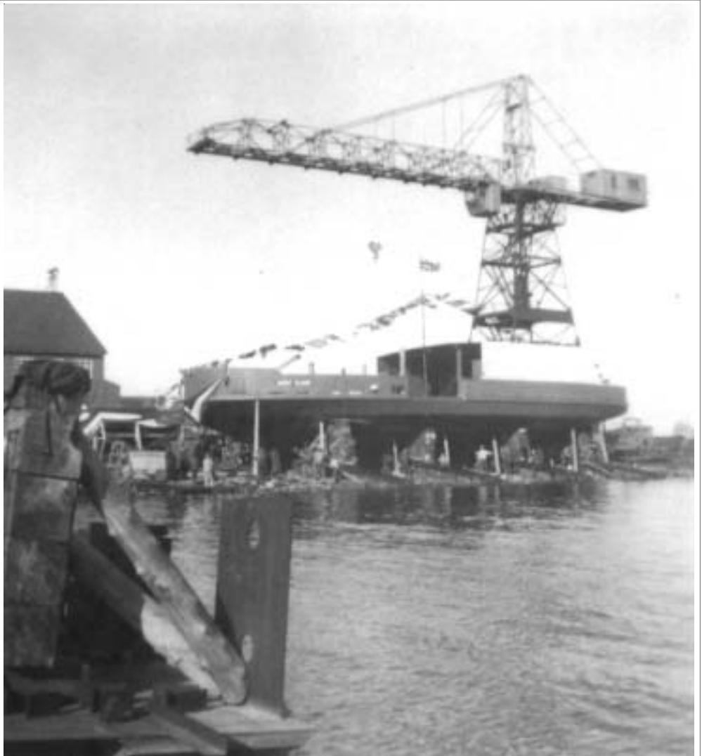
Construction and Launching of the MV Amherst Islander in 1955 (more on next page) Photo by Garnet McDonald
