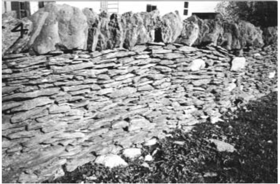
Stone Fence at Hazel DeHaan's house
